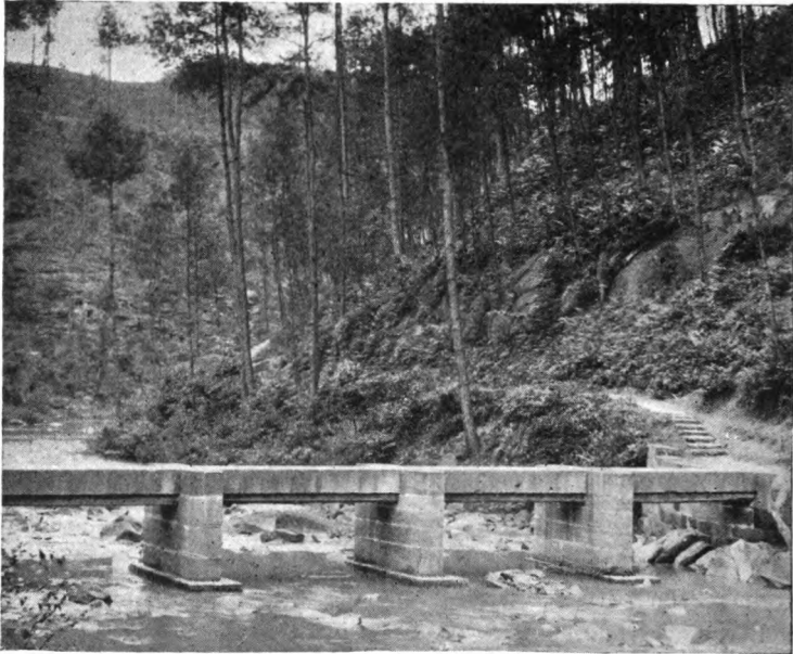
ONE OF CHINA'S BRIDGES.
